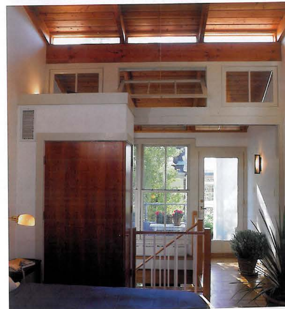
Large third-floor windows help to light the lower floors. An open stairwell channels sunlight from the top floor to the rest of the house. Sliding doors hidden behind the closet at left provide privacy for the bedroom. Photo taken at C on floor plan.
