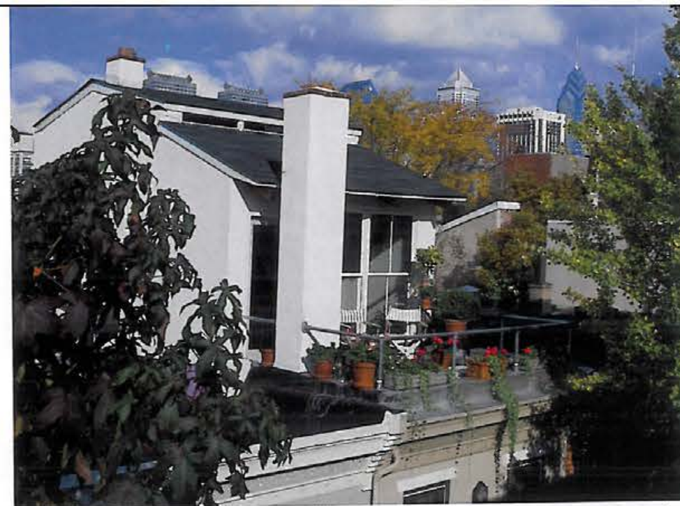
A third-floor addition gives the house extra room, light and a skyline view. The author designed this third-story addition to step back from street sight lines in compliance with historic-district code and to give the owner a small deck. Photo taken at B on floor plan.
